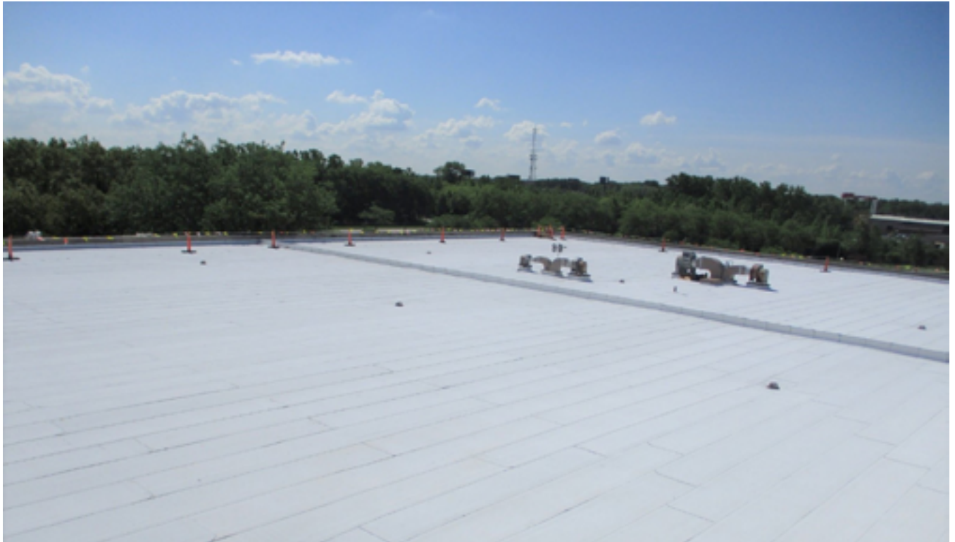
Roof replacement on District 6 (Markham) courthouse
