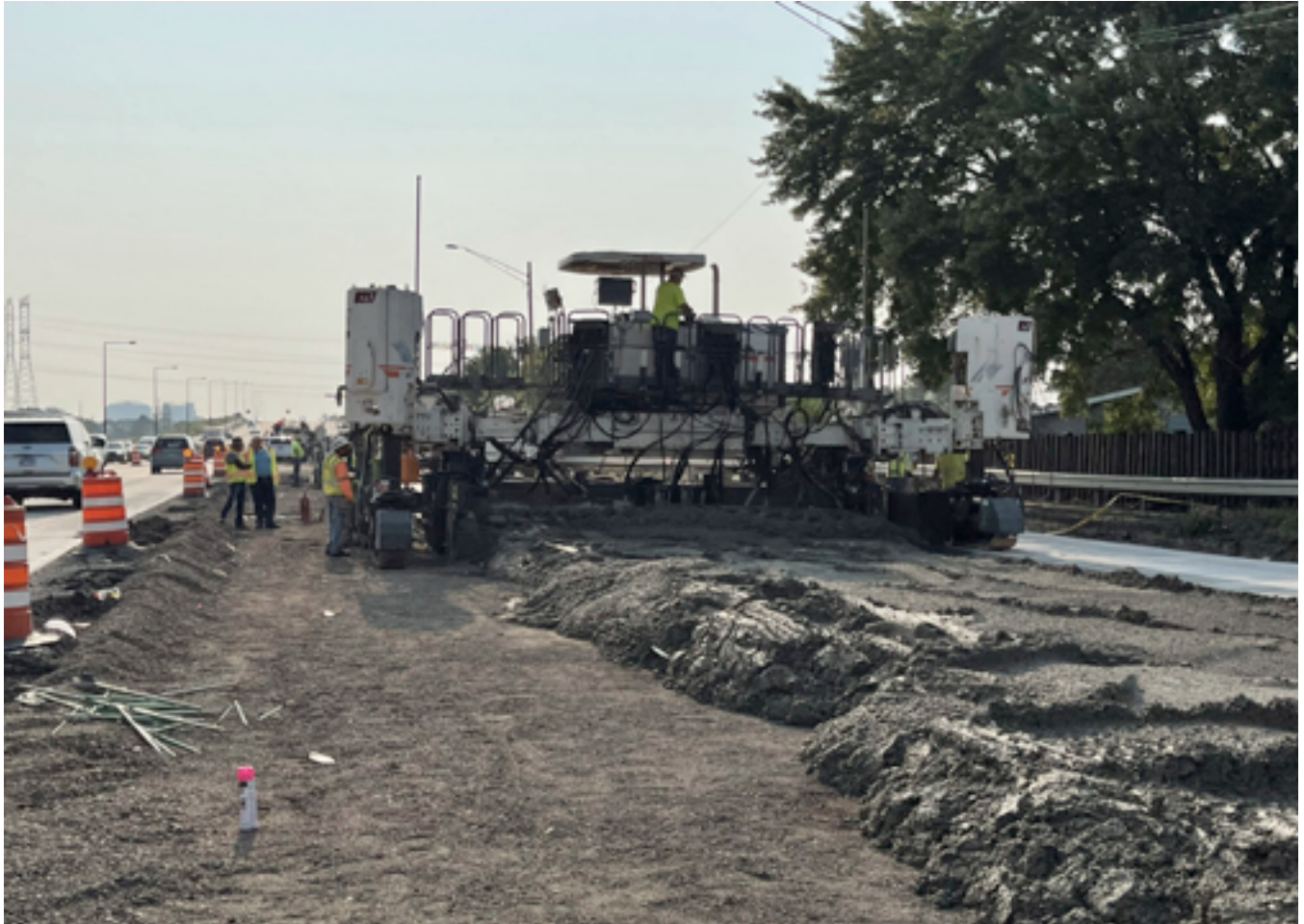
Figure 9: Cook County maintenance crews repair and maintain asphalt and concrete pavement surfaces. Existing asphalt surface was removed by milling, full depth deteriorated pavement areas were removed and patched with concrete, and the roadway overlaid with a new asphalt surface.
