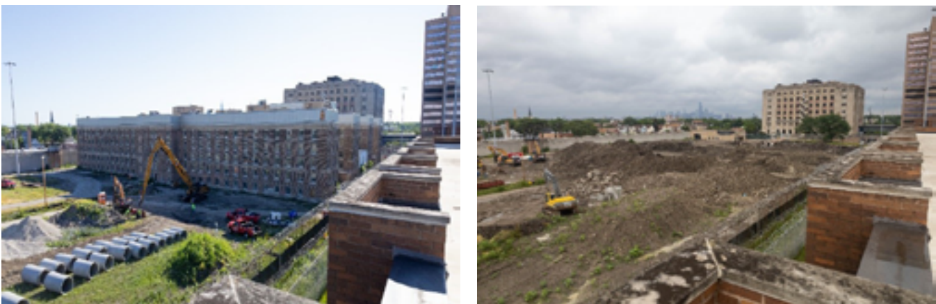
Before and After: the Demolition of Divisions 1 & 1A at the Department of Corrections Campus
