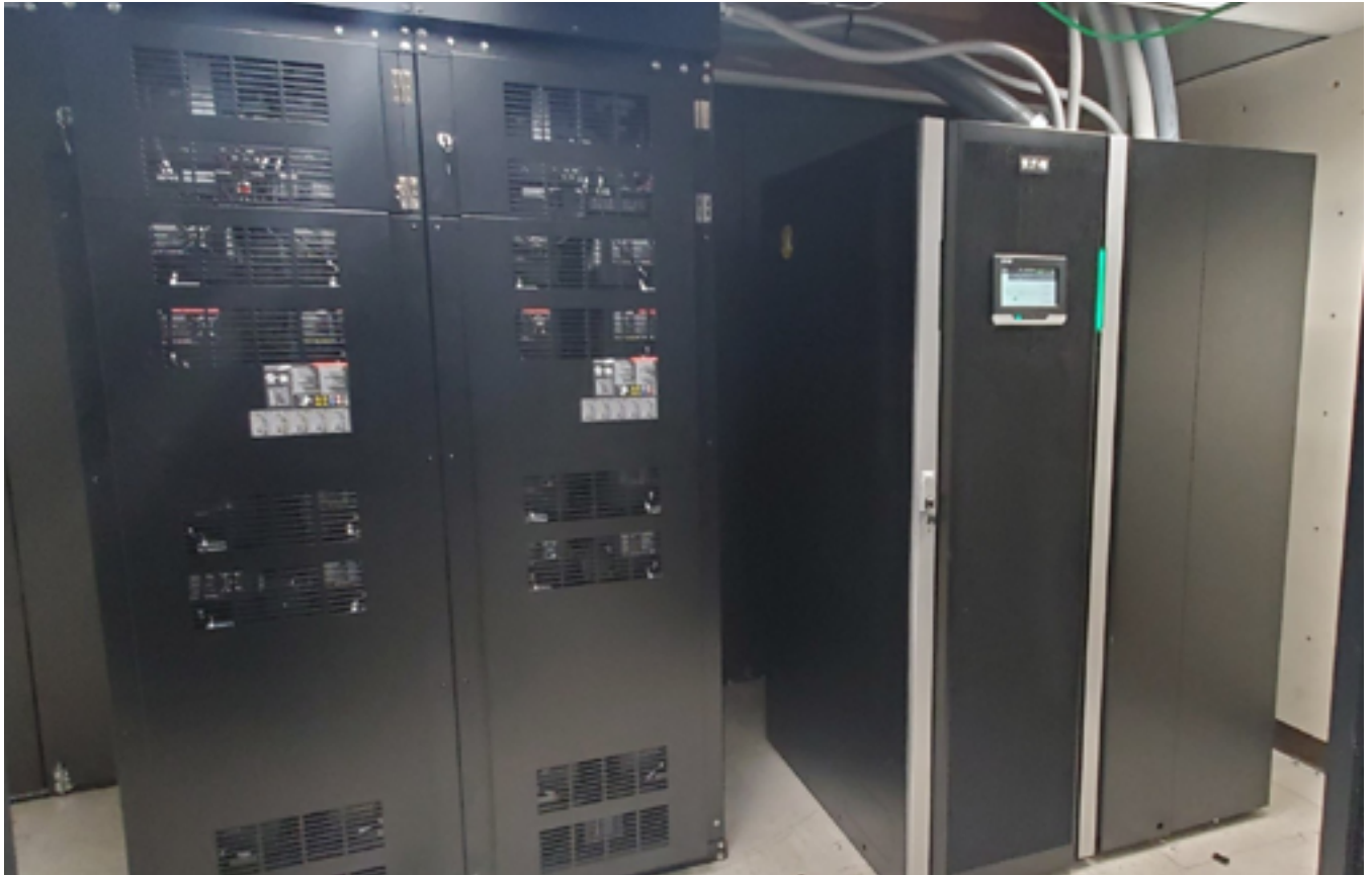
New UPS providing the necessary power redundancy for a County Server Farm
