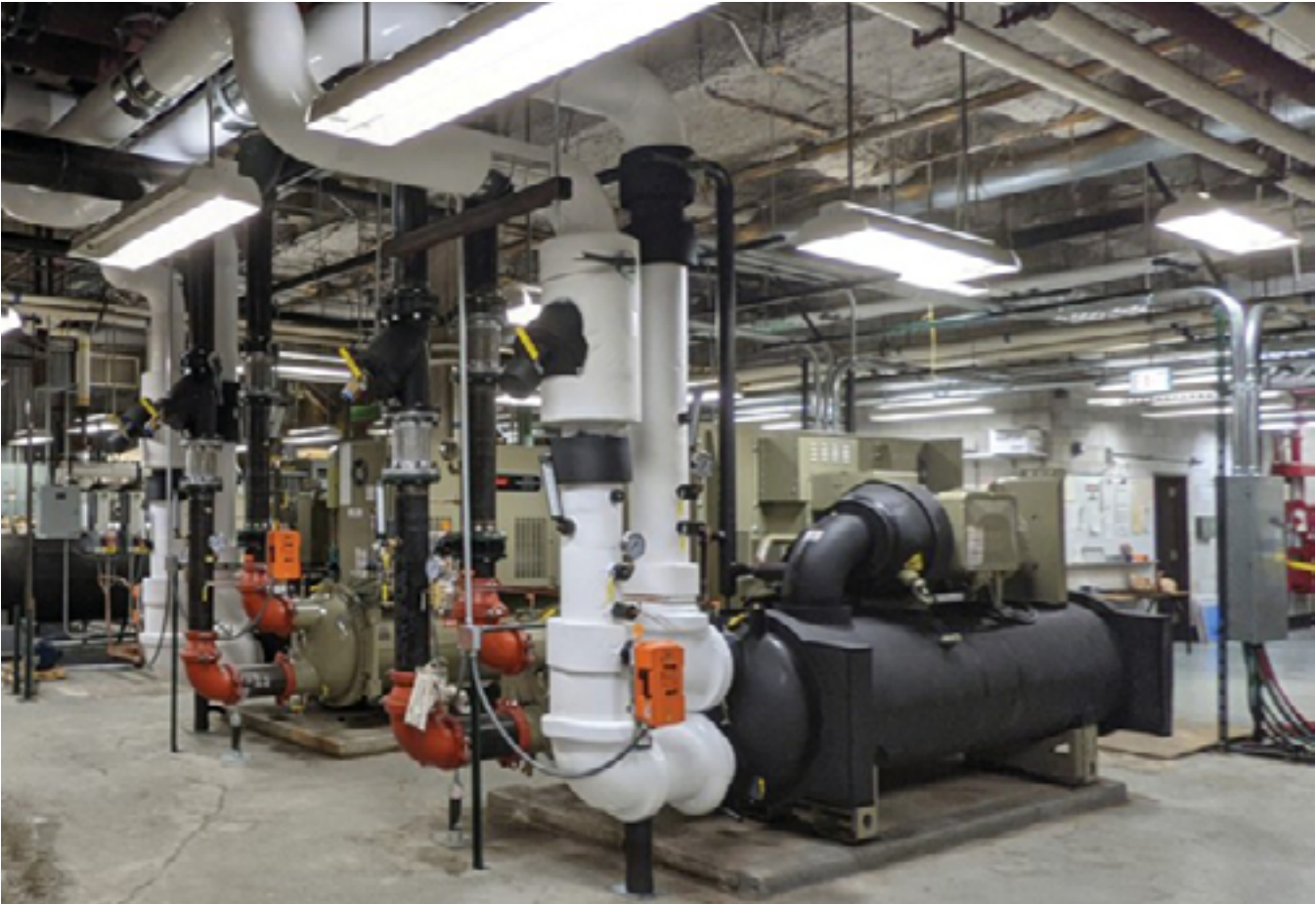
New energy efficient chillers at the Institute of Forensic Medicine
